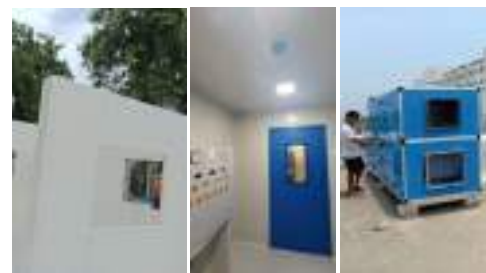
Installation of Panels & HVAC
